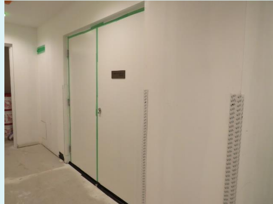
Figure 11- Electrical room temporarily sealed
