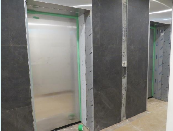
Figure 10- Elevators temporarily sealed at gaps
